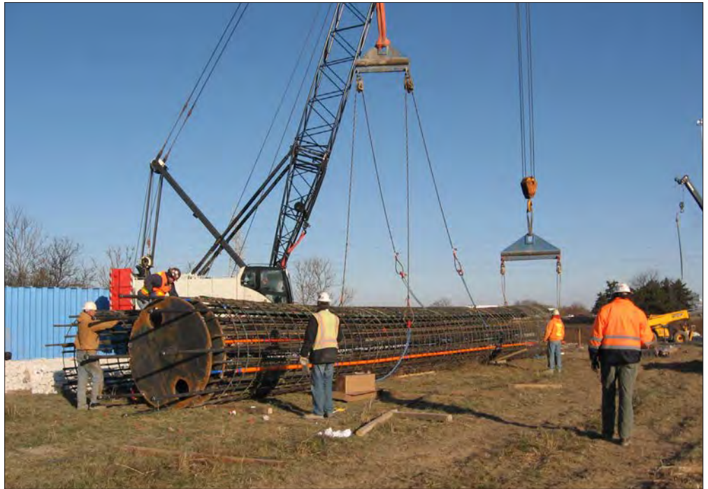
Crew assembling steel reinforcement for a drilled test shaft to determine the ability of the soil to support the Zoo Interchange bridges.
