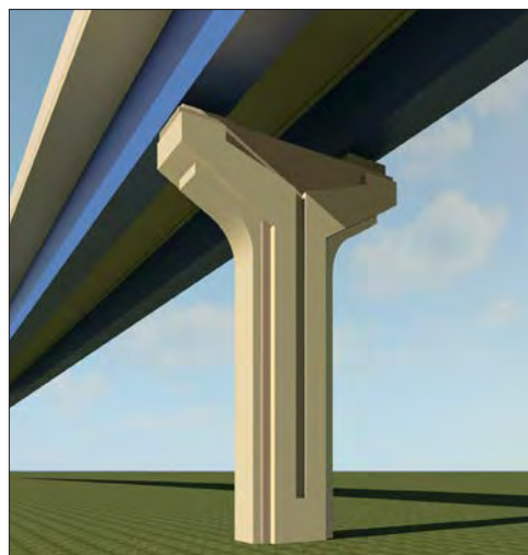
Typical pier structure for the core of the Zoo Interchange
