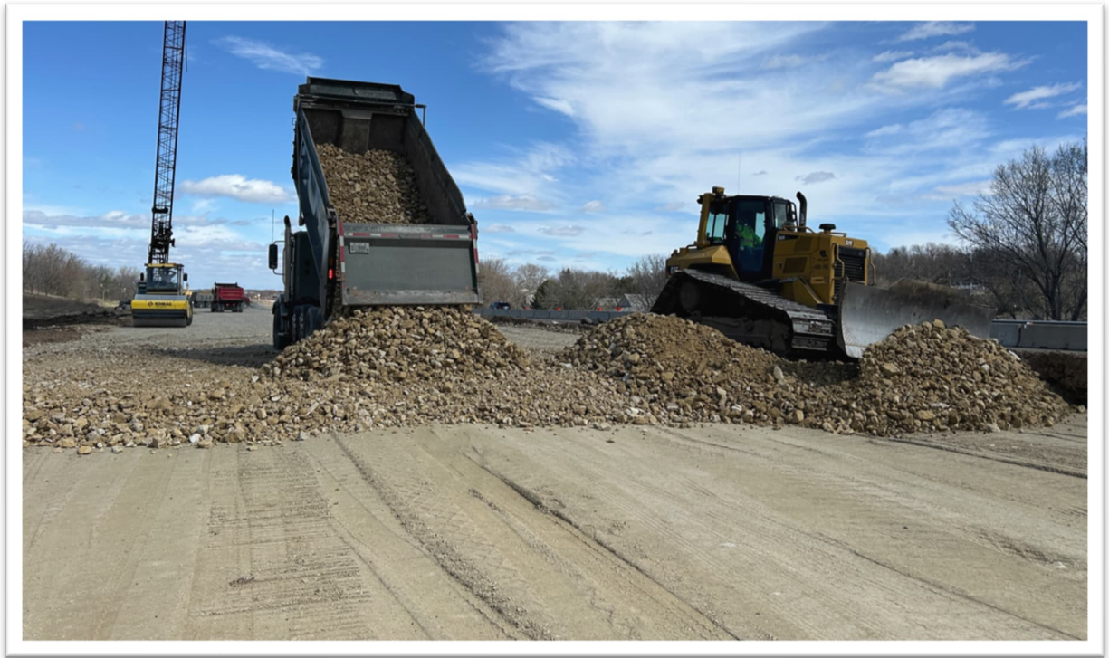
Placement of Aggregates Southbound USH 51
