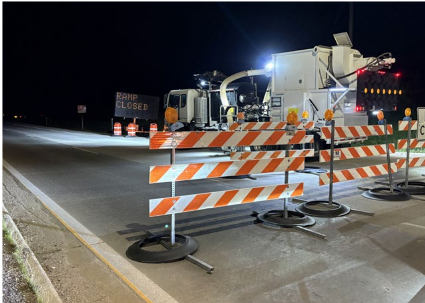
Above: Nighttime Pavement Marking
