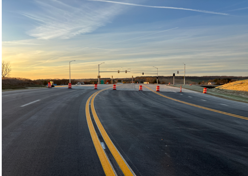
Above: Pavement markings and traffic signal poles along County G/Dairy Ridge Road
