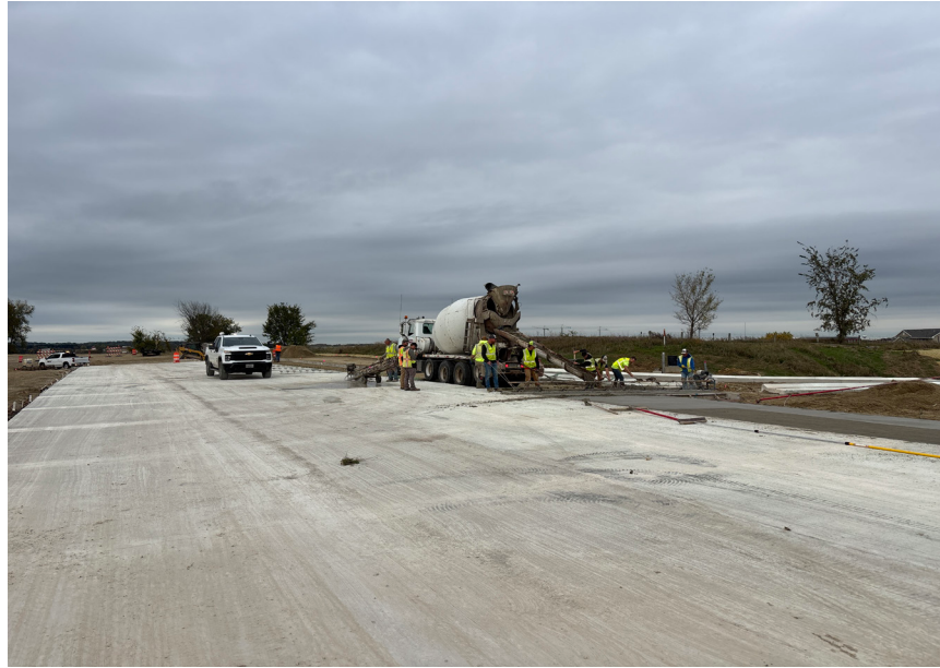
Above: Concrete paving on County G and Dairy Ridge Road
