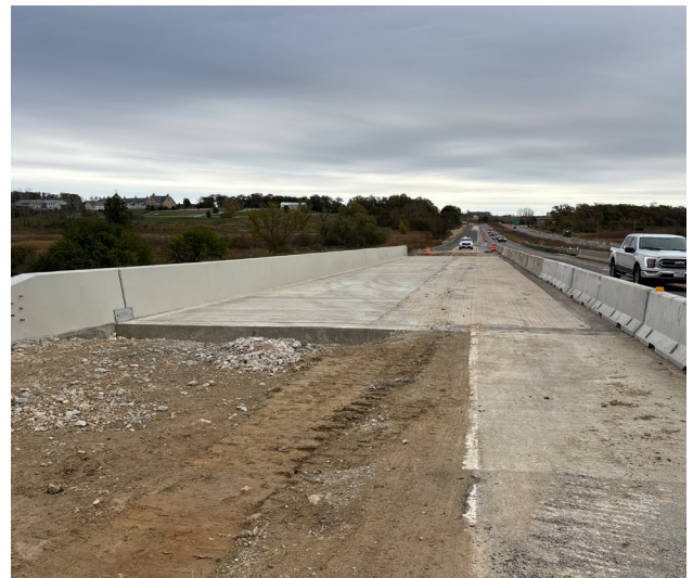
Above: Completed westbound Sugar River bridge widening
