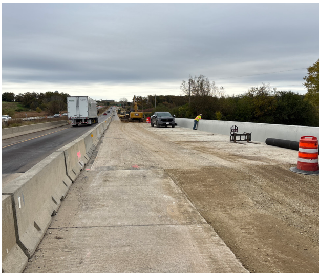
Above: Completed eastbound Sugar River bridge widening
