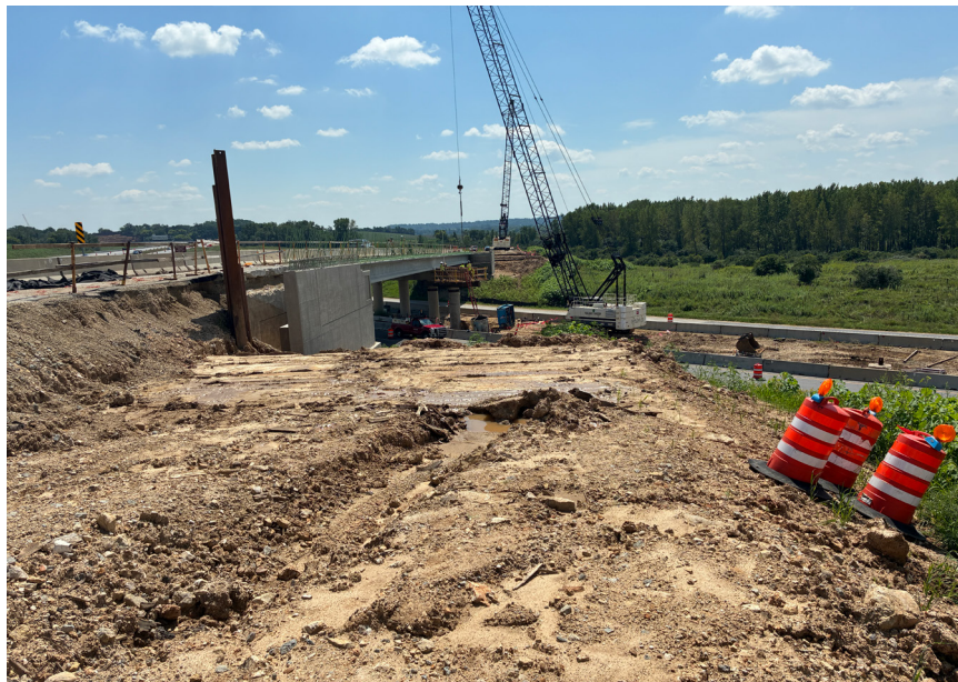
Above: Bridge widening pier construction along eastbound US 18 on-ramp
