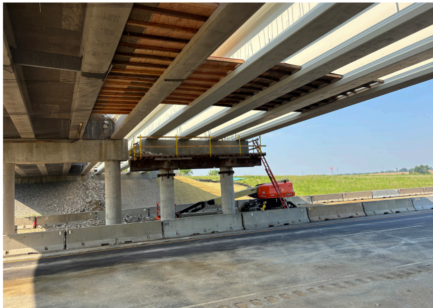
Above: Below County G bridge with girders in place and deck demolition in progress
