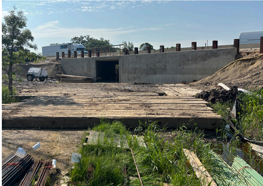
Above: Military Ridge Box Culvert north extension concrete work completed
