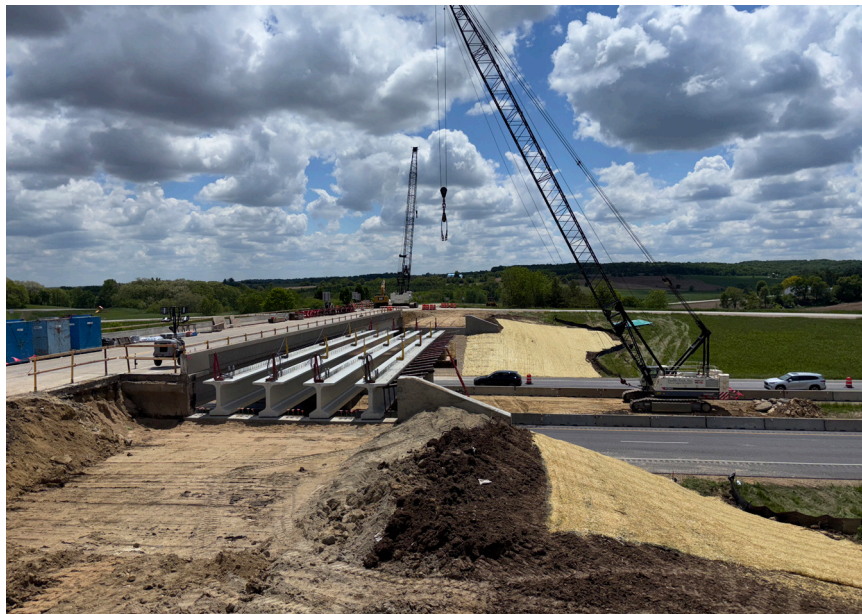
Above: Prestressed concrete girders set in place at County G bridge
