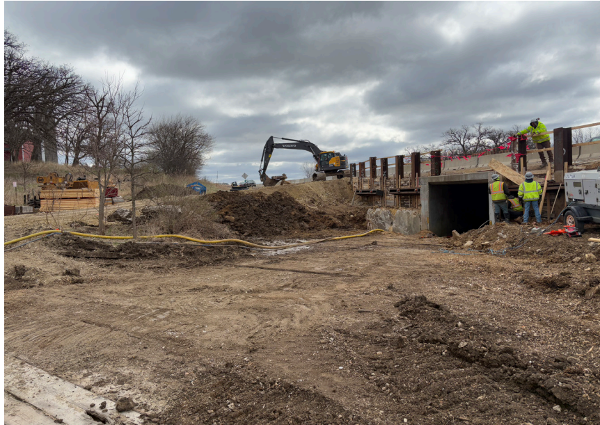
Above: Wing wall removal at Military Ridge Box Culvert north of US 18/151
