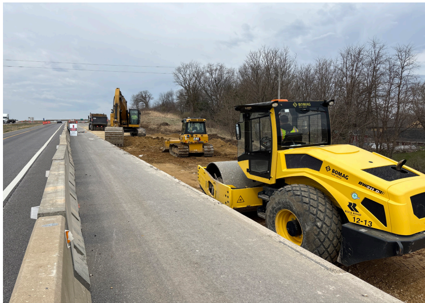
Above: Westbound US 18/151 auxiliary lane widening and grading
