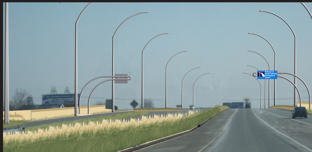
Curb & Gutter Treatment in Median
