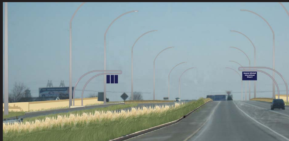
Curb & Gutter Treatment in Median
