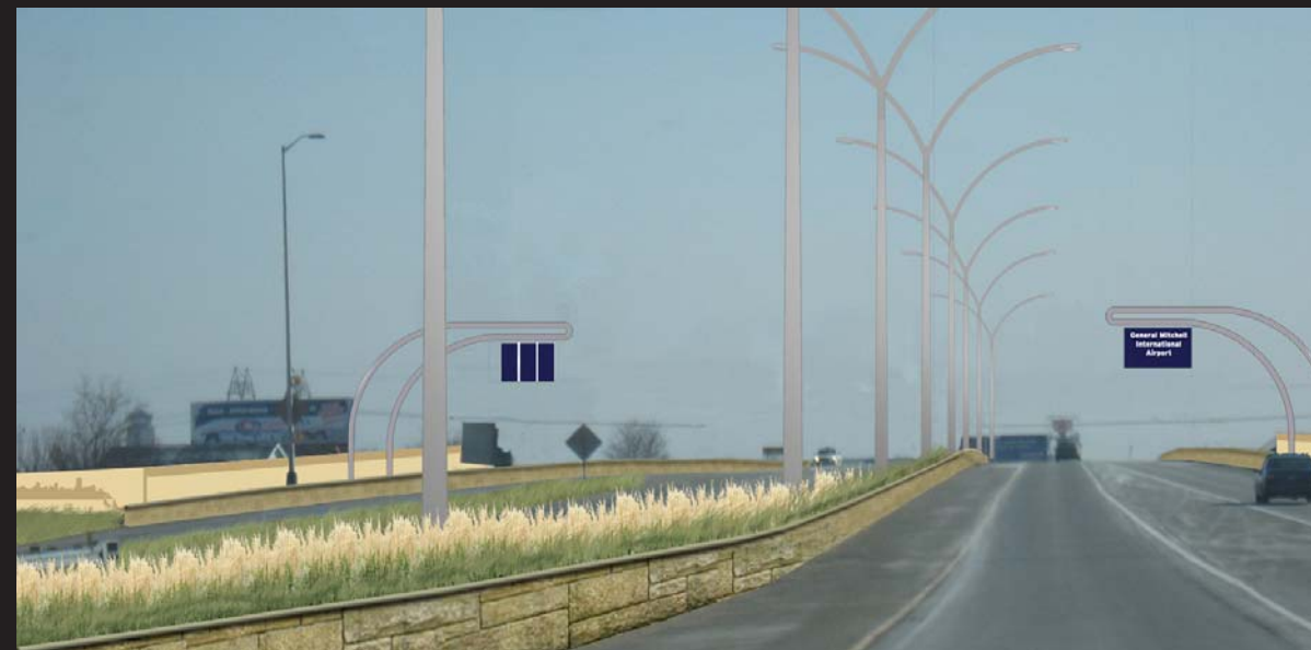
Retaining Wall Treatment in Median
