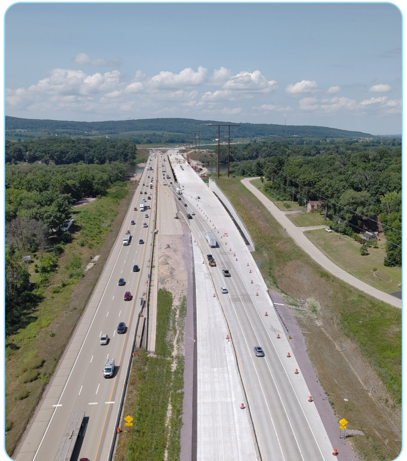
Above: The newly reconstructed northbound roadway and river bridge
