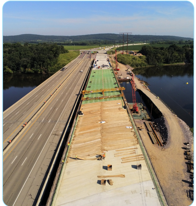
Above: Preparation for the final deck pour on the new northbound bridge
