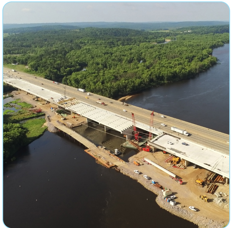
Above: Girder placement for the new northbound river bridge
