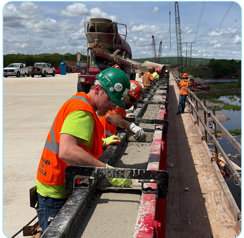
Above: Parapet construction for the new northbound river bridge
