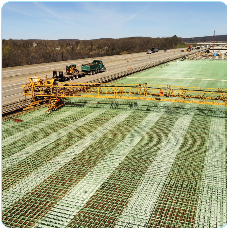
Above: Steel reinforcement for the new northbound river bridge
