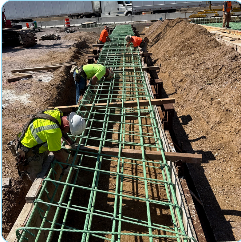
Above: Steel reinforcement for the new northbound river bridge approach
