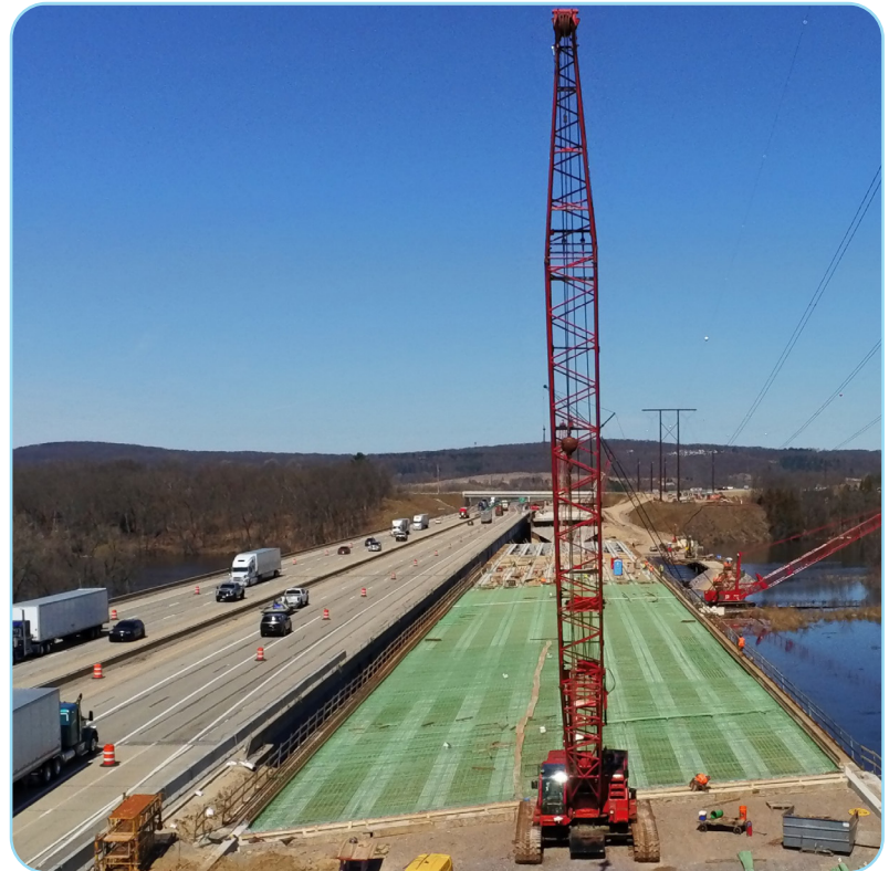
Above: Bridge construction for the new northbound river bridge
