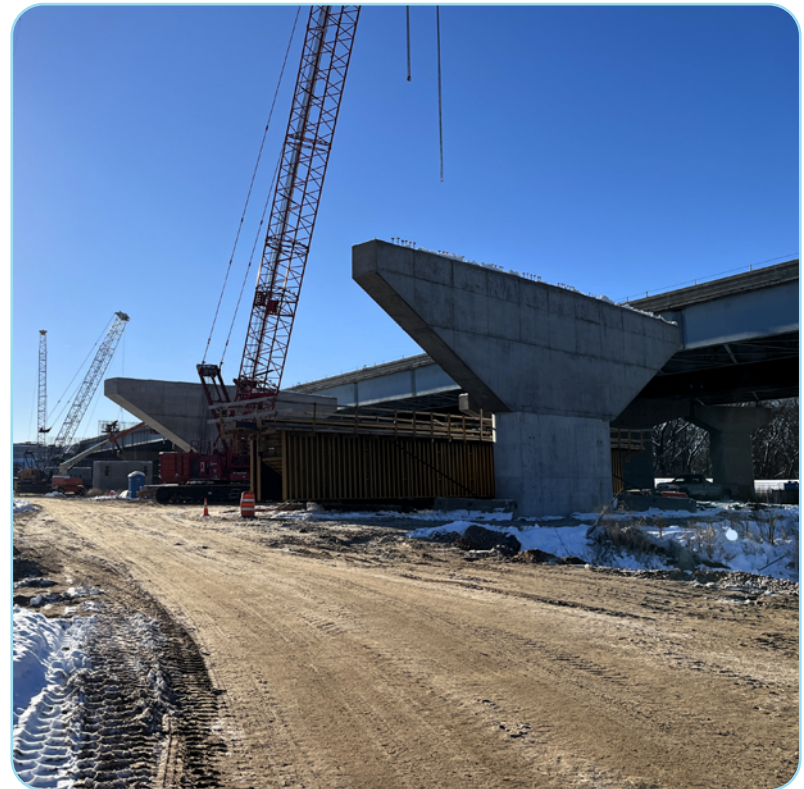
Above: Ongoing pier construction of the new northbound river bridge
