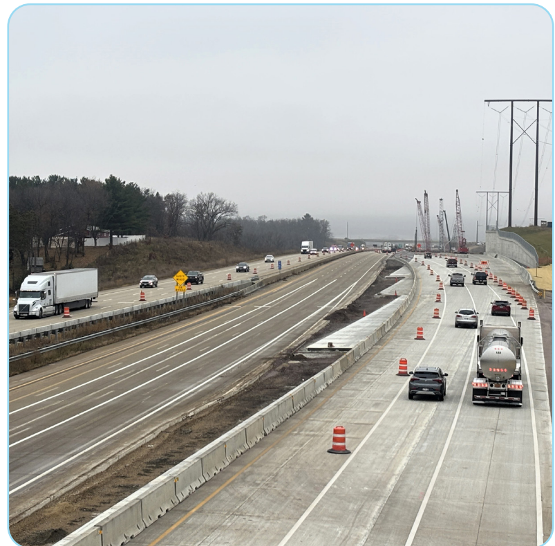
Above: I-39/90/94 Northbound (WB) traffic shifted to new concrete pavement
