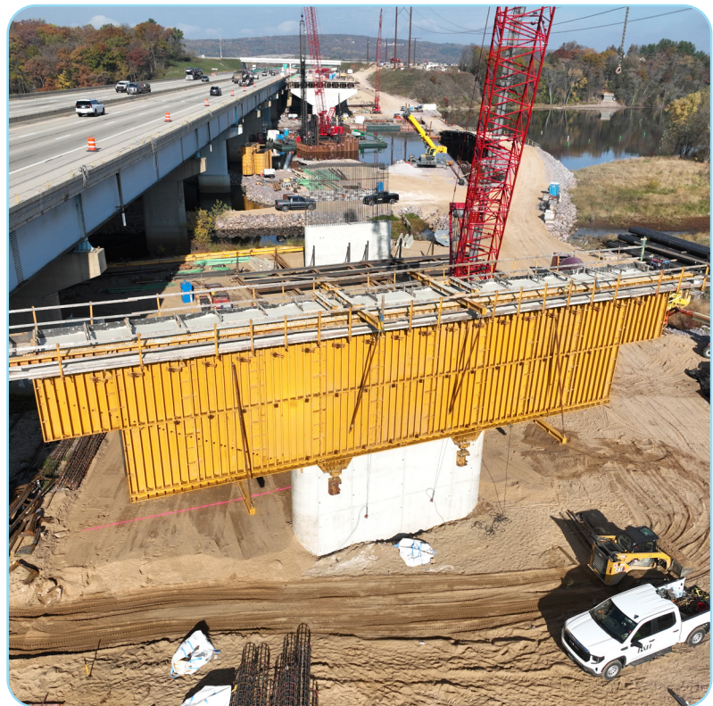
Above: Pier construction for the new northbound river bridge
