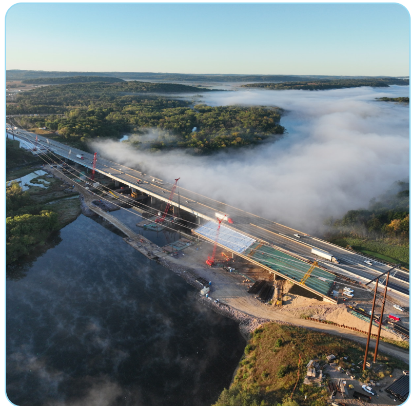
Above: The new I-39/90/94 northbound river bridge
