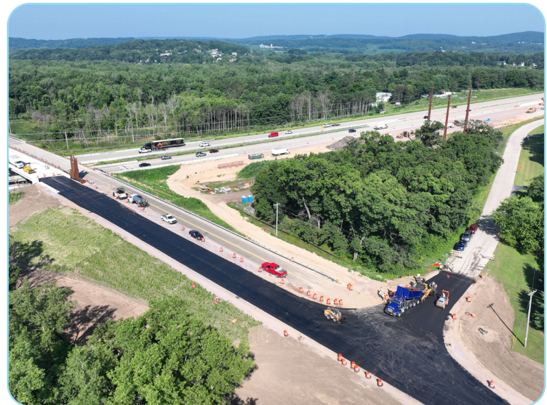
Above: Asphalt paving for the new County V roadway
