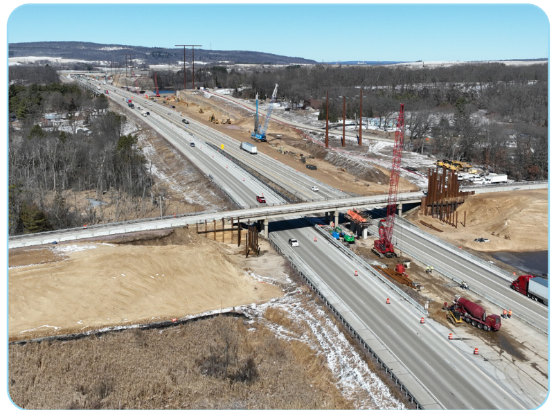
Above: County V over I-39/90/94 facing north
