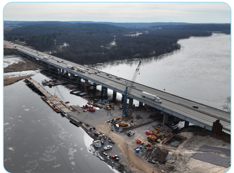
Above: I-39/90/94 facing southwest
