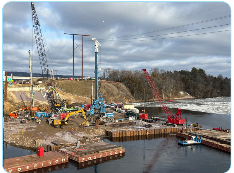
Above: Wisconsin River Bridge causeway
