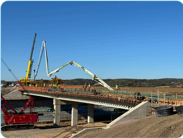
Above: County U bridge construction over I-39/90/94
