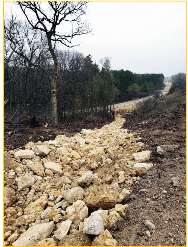
Comprised of varying sizes of rock, riprap is used to prevent erosion from rainwater, typically along hillsides and embankments.
