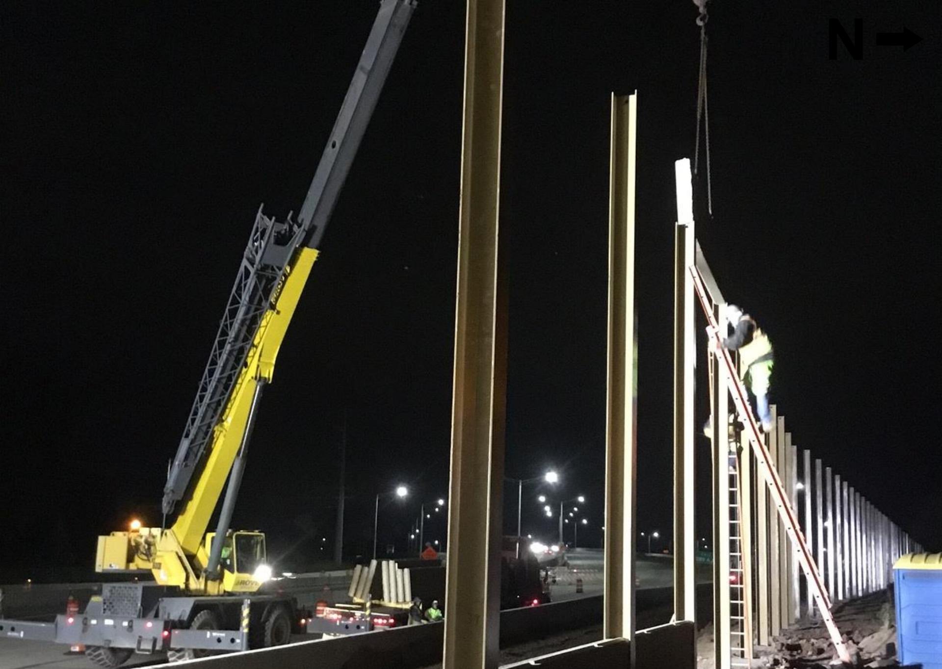
Noise panel installation along Racine westbound exit ramp
