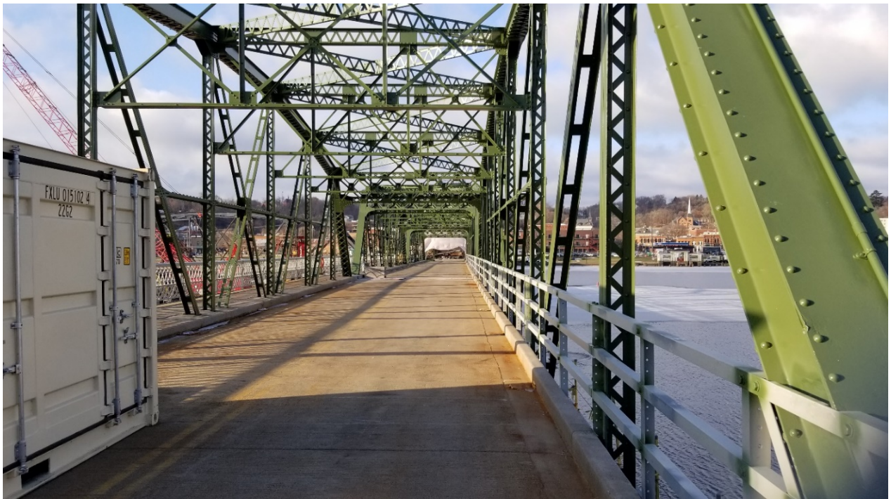
View of painted lift bridge trusses
