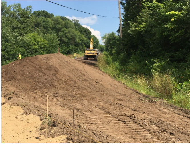
Looking East at the removal of asphalt along the old County E corridor and restoring to a naturally vegetated state.
