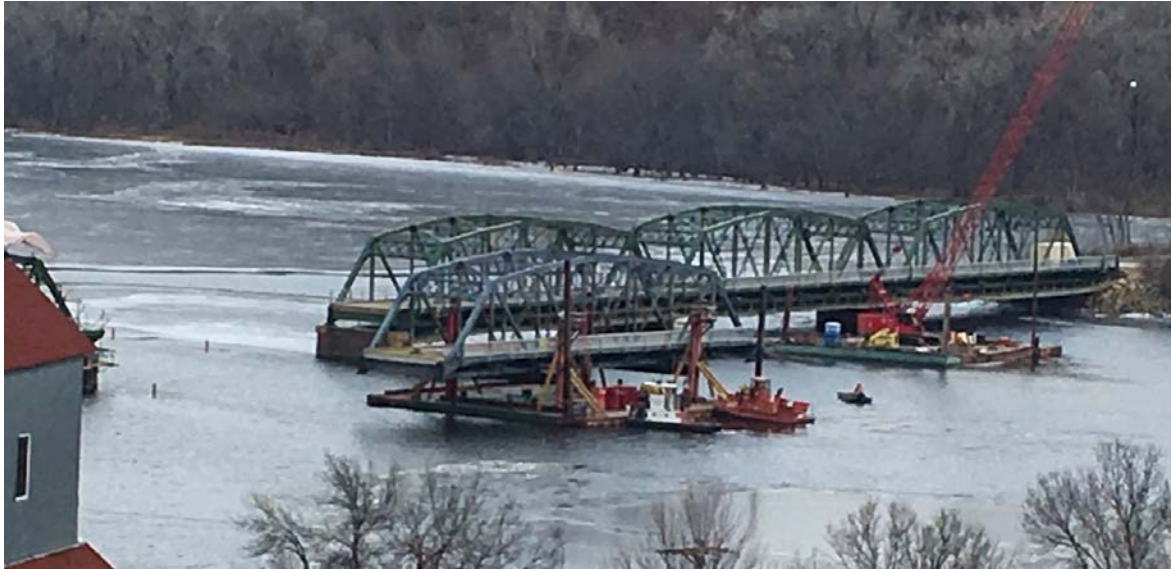
View of Lift Bridge from MN bluff – Span 6 being replaced
