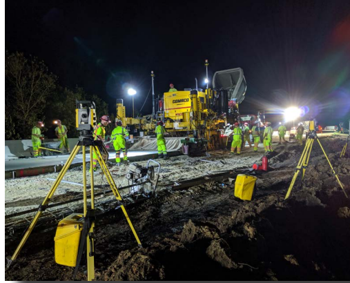
Crews built concrete crossovers south of the I-39/90 and US 12/18 (Beltline) interchange to accommodate future traffic staging. In 2020, the Interstate will be expanded to three lanes each way from County AB to the Beltline interchange.
