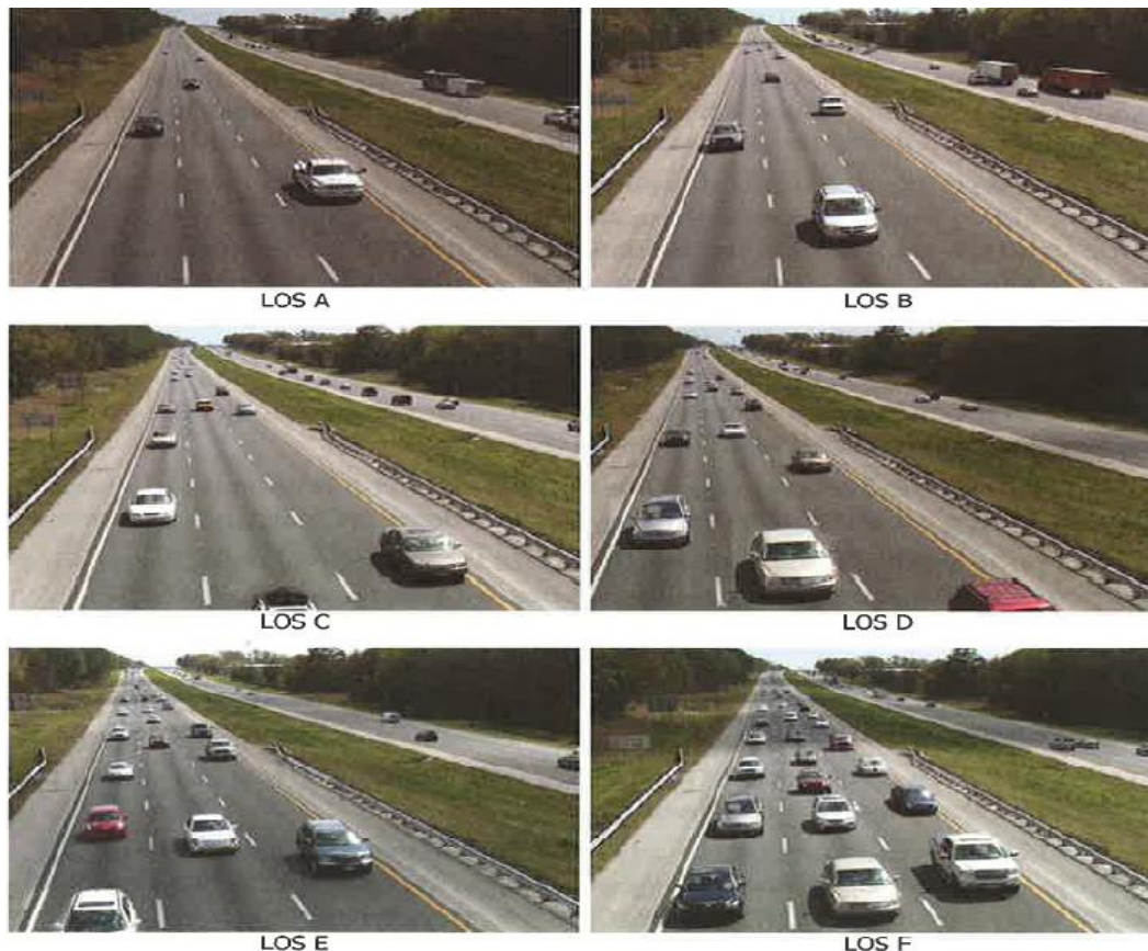
Figure 6 - Level of Service Characteristics 7
