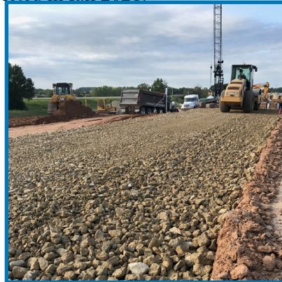
(Left) Construction continues this summer on the new I-39/90 northbound bridge over the northbound Interstate ramp to westbound US 12/18 (Beltline) in Madison. (Center) Crews placed the first area of select crushed aggregate for the new subgrade as part of the I-39/90 and US 12/18 (Beltline) interchange (Exit 142 A-B) reconfiguration in Madison. (Right) Crews continue reconstruction and expansion of I-39/90 northbound between County AB and the US 12/18 (Beltline) interchange near Madison.
