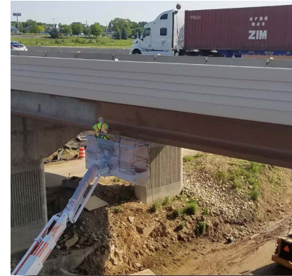
A crew member applies stain to the bridge girder as work winds down on the Rock River bridges replacement project.
