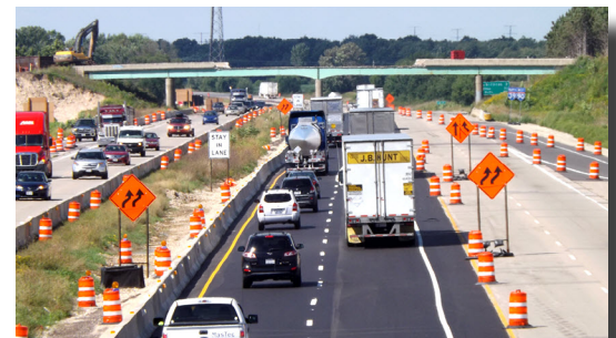
Motorists use temporary widening on I-39/90, north of WIS 59, as crews reconstruct the new northbound Interstate lanes in this area.
