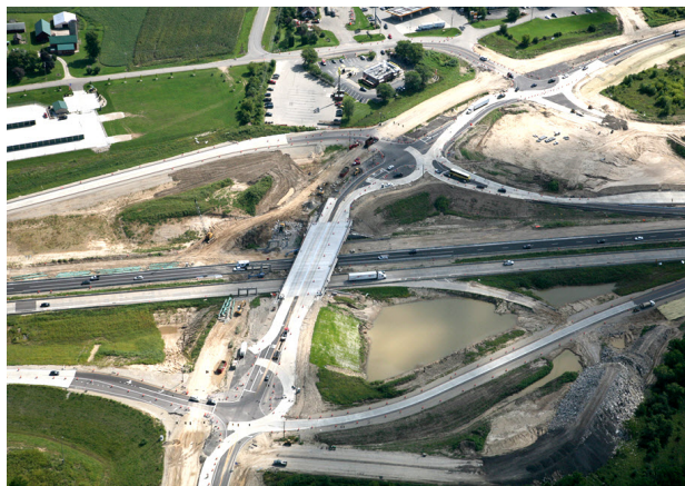
The three roundabouts begin to take shape, as work progresses on the I-39/90 and WIS 59 interchange in northern Rock County.
