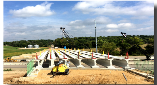
The County BN bridge over I-39/90 is removed and lengthened to accommodate future Interstate lanes.
