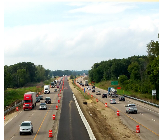
Temporary widening occurred on I-39/90 southbound near Edgerton this year. All Interstate traffic will be shifted onto this side next year during the I-39/90 northbound expansion in this area.
