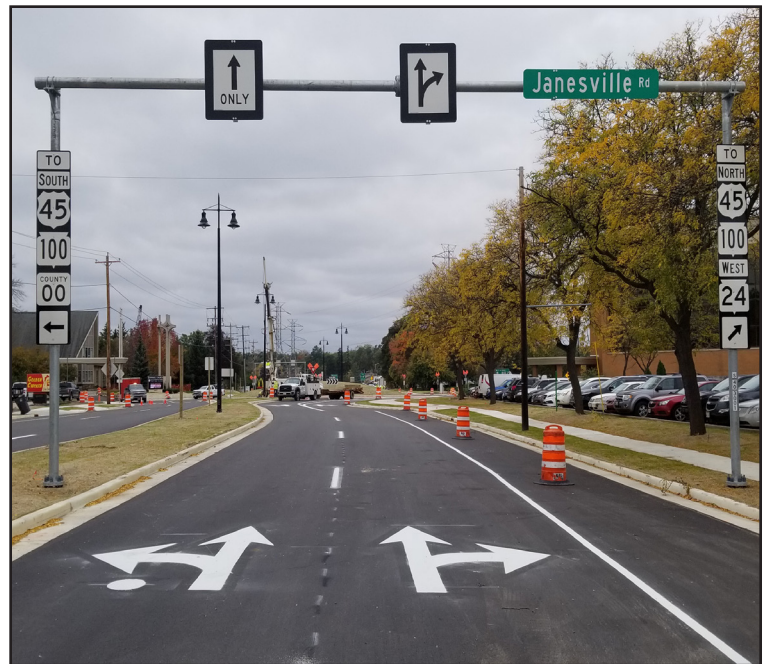
Overhead sign structure approaching roundabout
